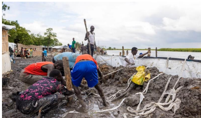
Figure 6. Simple but effective reinforcement of the dikes, which prevented the flooding of Old Fangak.
