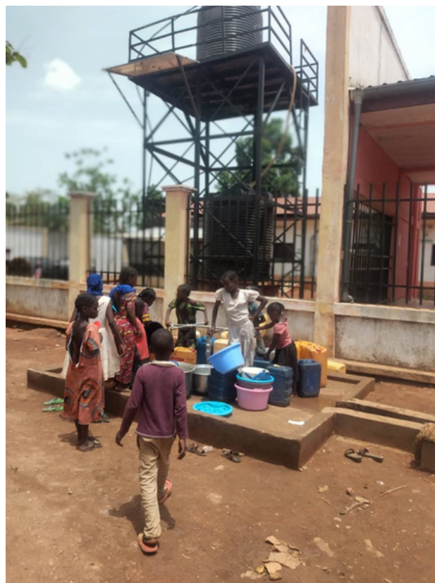
Picture from Arsene Nabeje Description: Neighboring inhabitants of Elevage Health Centre near Bambari, CAR, taking water from a tap stand supplied by a solar system dispensing safe water to both the public and the health center.
